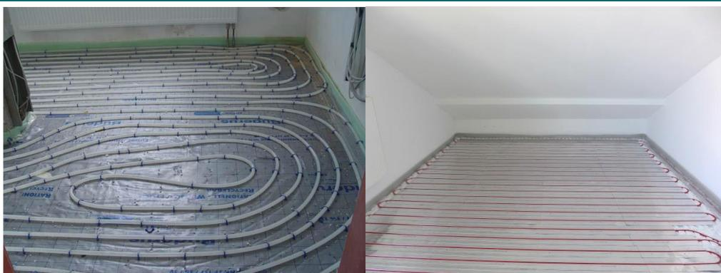
Figure 24. Spiral pipes of the dining room in the ground floors (left) and the child 2 rooms' serpentine pipes in the attics' (right) underfloor heating during installation.
