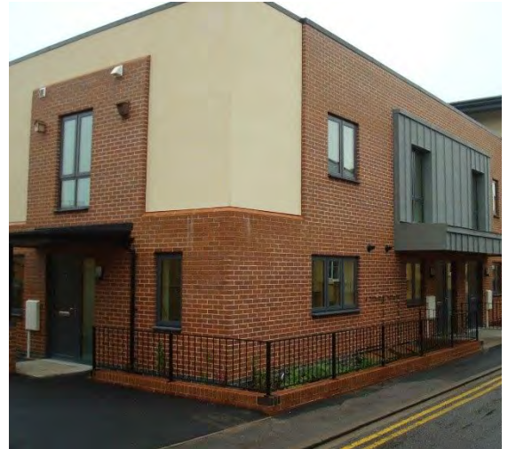
View on the South end of the CE1 test case building
