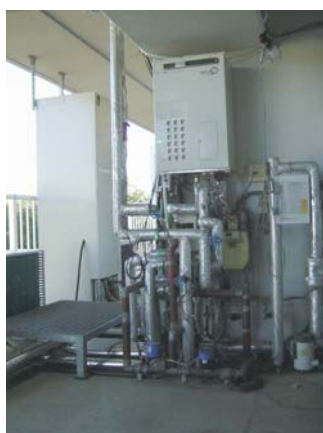
Boilers and CO 2 heat pump system for DHW: Efficiency of several heat sources is measured with changing connection between the heat source and piping dwelling unit.
