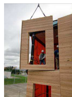
Wooden façade element, developed together with Biohaus Goierri, S.L.
