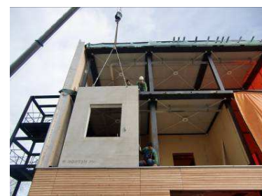
Prefabricated concrete façade element, developed with Norten-pH
