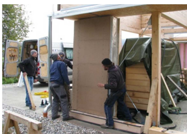
Mounting of wall assemblies
