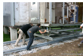
Rail system for placement of the movable Coldbox.
