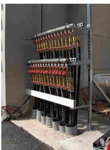
Manifolds connected to the ground heat exchangers
