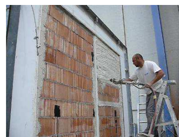
Insulating mortar projection.
