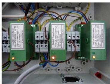
Electrical transducers for heat pump (one for compressor, one for ground heat exchanger pump and one for heating floor pump)
