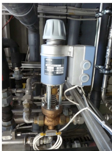
Electromagnetic 3-way valves for temperature controlling
