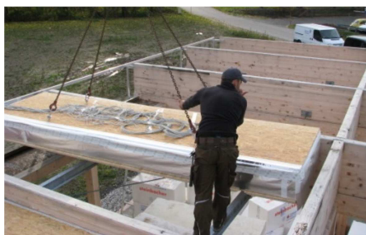
Mounting of roof assemblies
