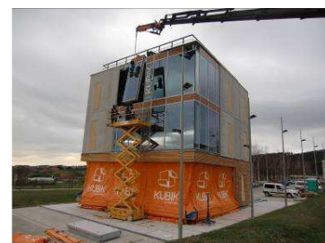
PV-Curtain wall developed by TECNALIA
