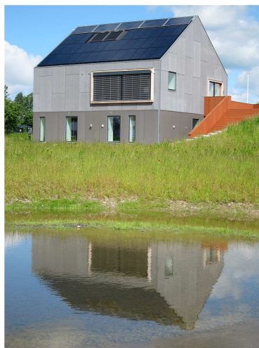
Optimized control of e.g. solar screening in order to decrease overheating.
