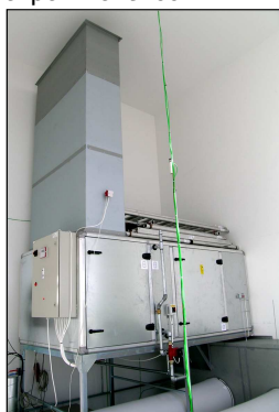
Ventilation system in the experiment room
