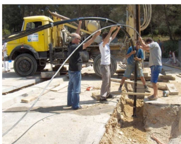
Implementation of a double-U heat exchanger in the ground
