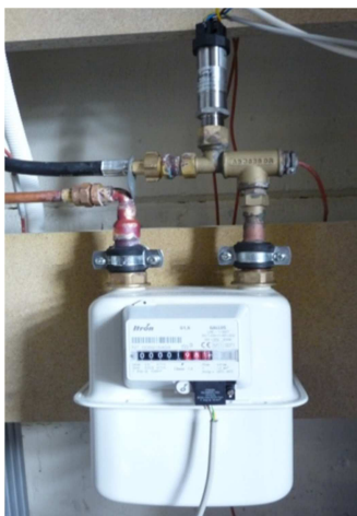
Gaz counter and pressure transduce
