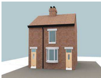
The Energy House and its adjacent conditioning void, used to control and monitor energy loss and heat transfer through party walls.
