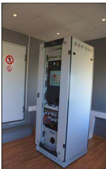
Rack mounted computer and data acquisition system in the service room of a test cell.
