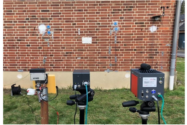
Setup for wall surface temperature/U-value measurement using different types of infrared cameras
