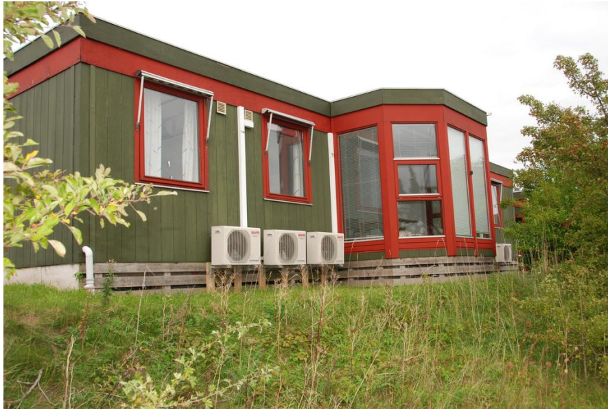
Figure 10. Experimental FlexHouse at RISØ in Denmark
