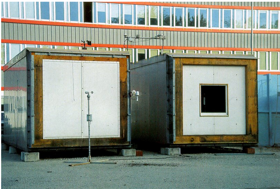
Figure 1. Homogeneous opaque insulated panel and a simple window system placed in the south wall.
