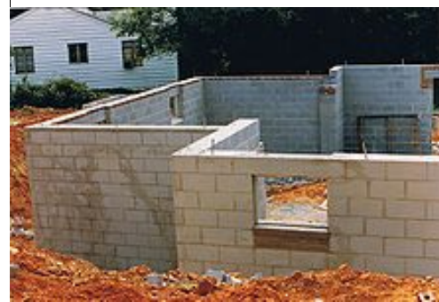
Figure 2. Building wall under construction
